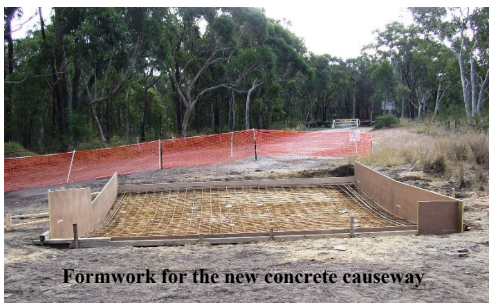
Ground being prepared for the new causeway
